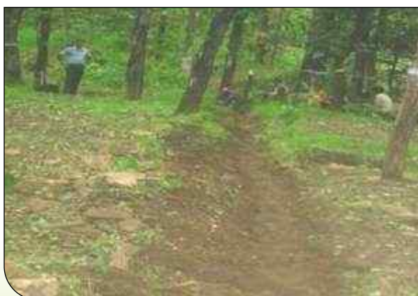
Trench around the plot
