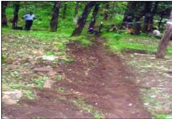
Digging of Trench around the plot
