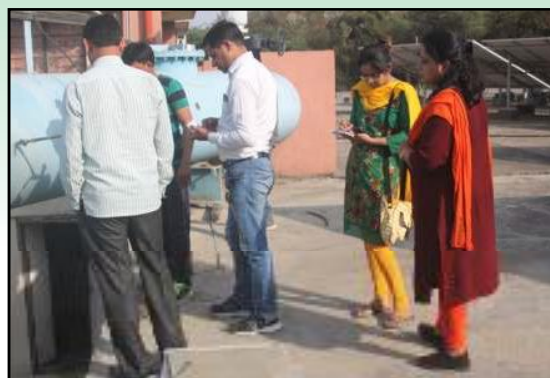
Ramnagra Treatment Plant
